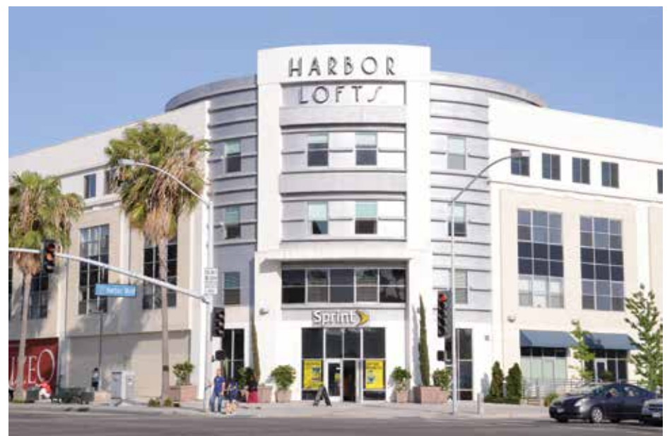
Harbor Lofts features a 3,000-square-foot ground-floor retail property with three levels of residential lofts, townhomes and condominiums above.
